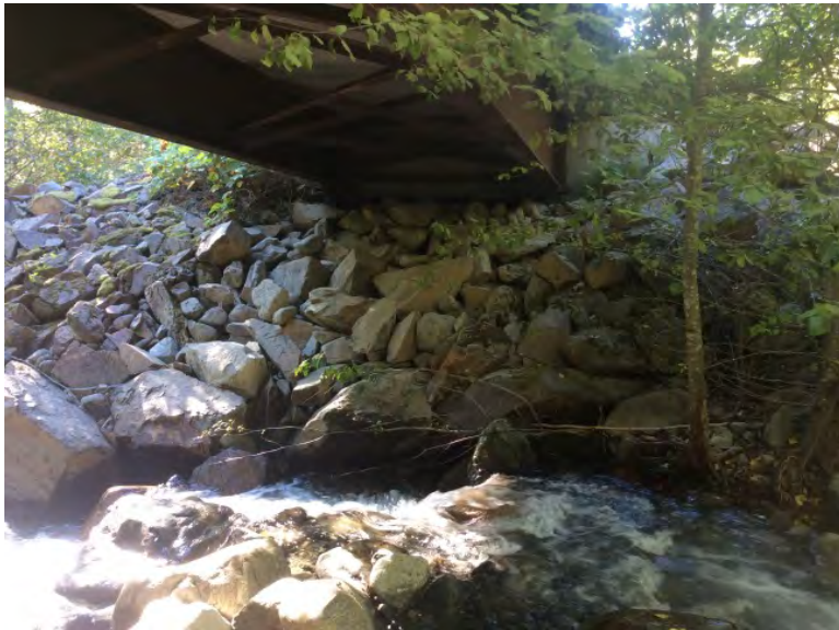
Right Bank Abutment when facing downstream
