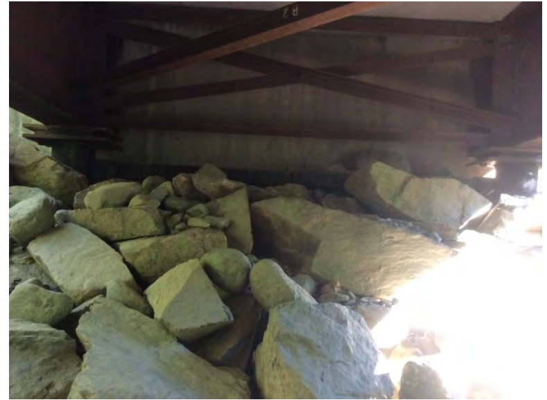
Left Bank Abutment when facing downstream
